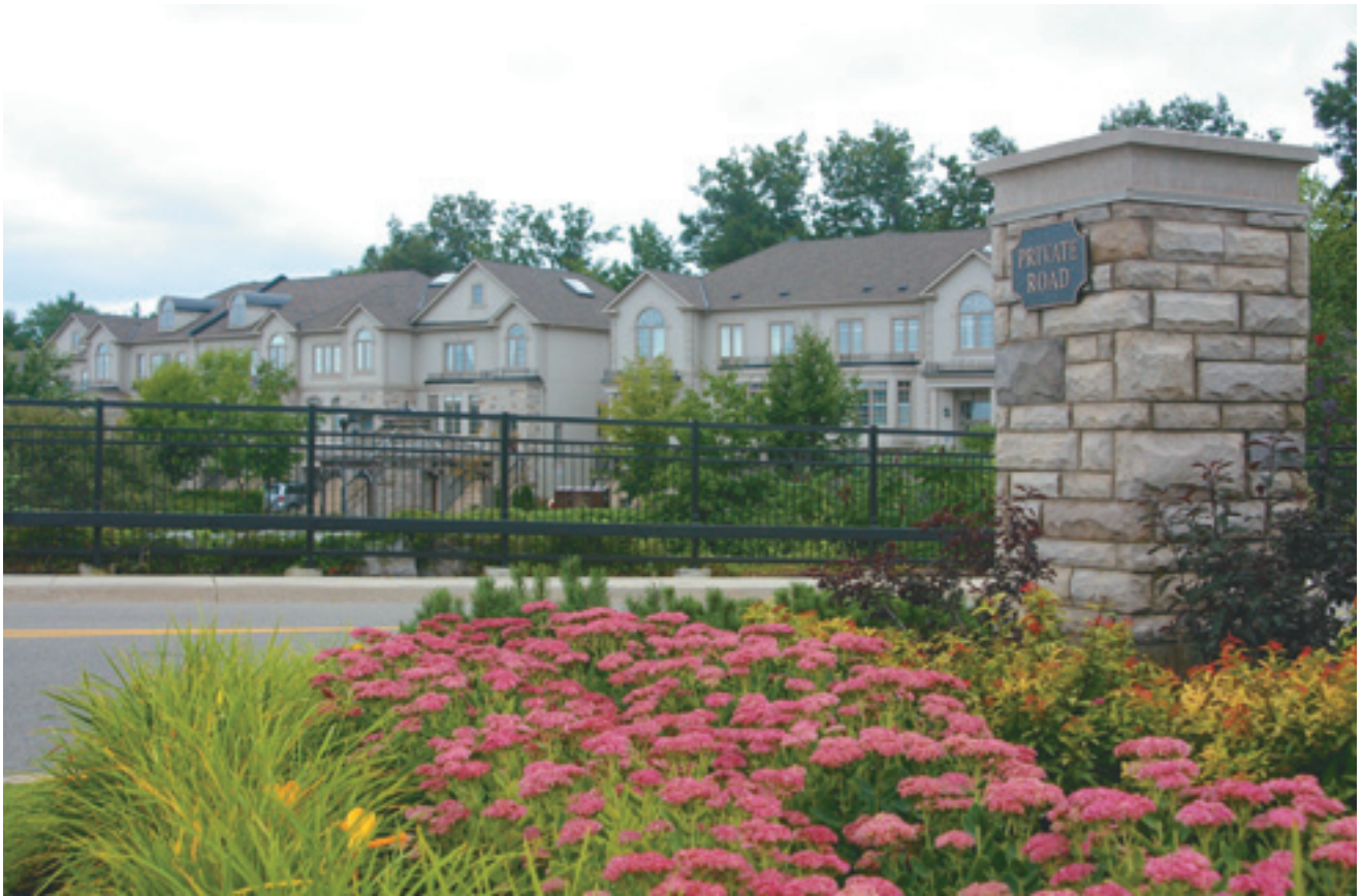
High-end condominium with perennials and a drainage collection pond.
